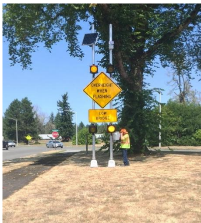
Warning Sign with Flashing Beacons & Audible Horn:
